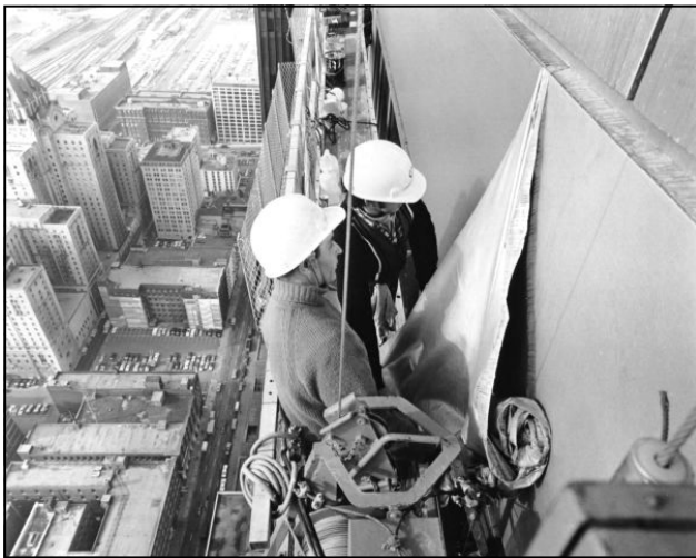
Commerce Court under construction
